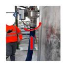
the Driver connects his own flexible hose to the tanker, then connects the other end to the silo pipe by turning counterclockwise
